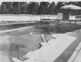
IN THIS over-all view of the model basin is the measuring bridge with instrumentation for recording swell movement. DEN E vista total aki di e basin di modelo tin e brug di registracion cu instrumentacion pa midi e movimiento di marea.
